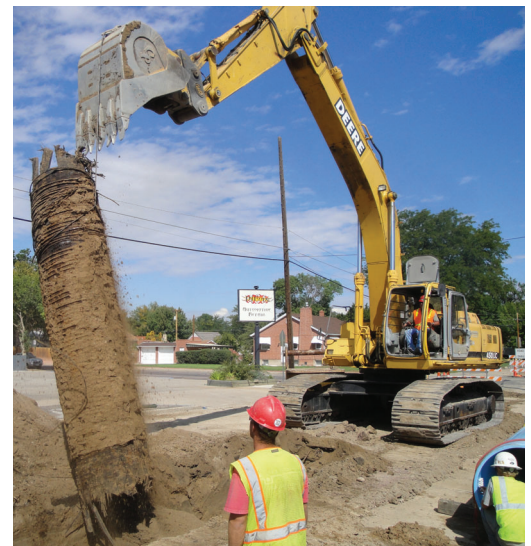
Removal of last wooden main line
