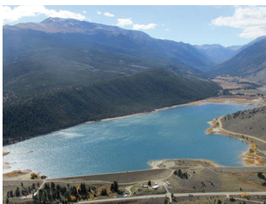
Clear Creek Dam and Reservoir
