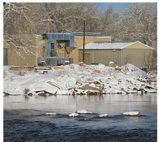
Winter at the Comanche pump station
