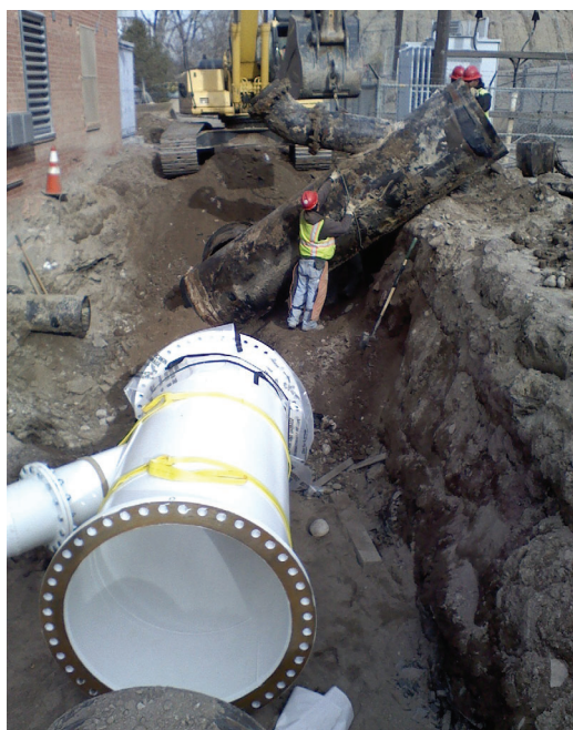
Replacing main lines
