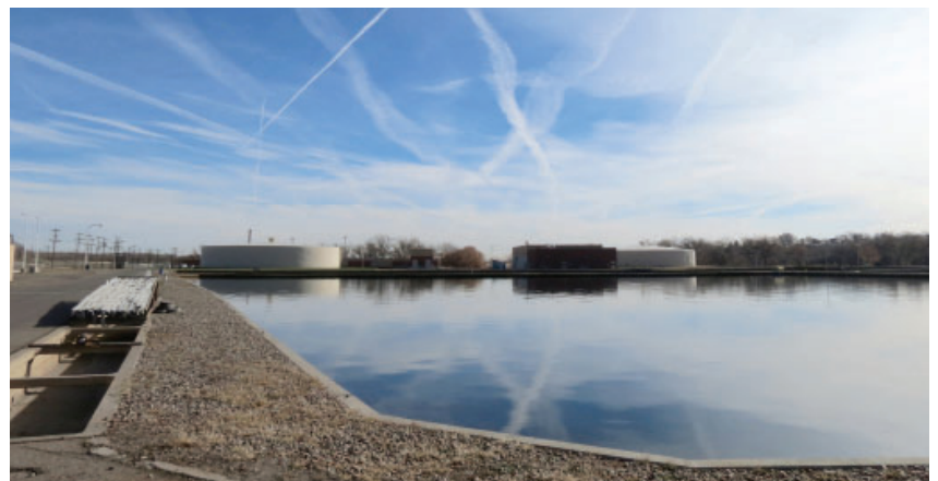
Settling pond at Whitlock Treatment Plant
