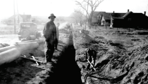
Installing water mains
