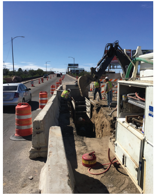
Replacing main lines
