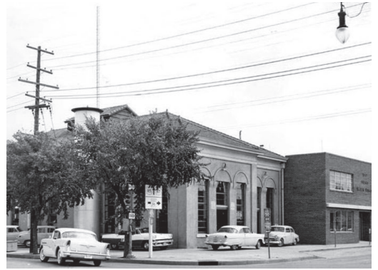
Pump house and offices, circa 1950s
