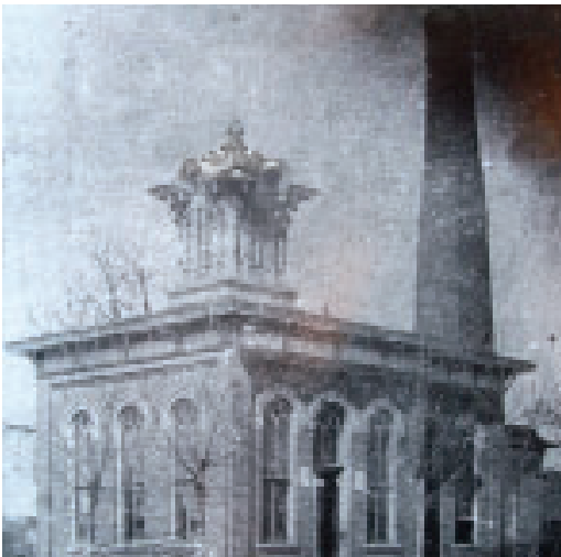
Original pump house at 4th & Grand Ave.
