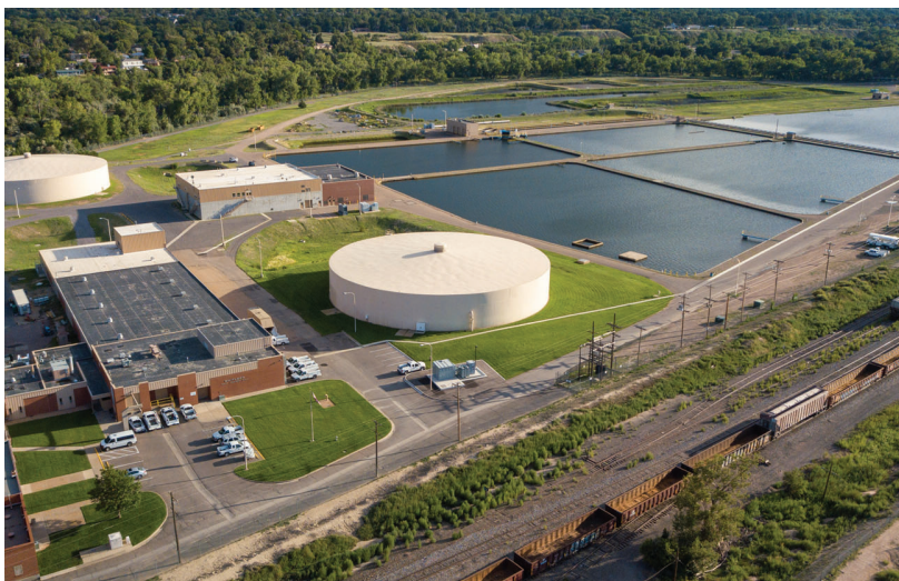
Whitlock Treatment Plant
