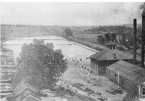
Southside reservoirs and pump house
