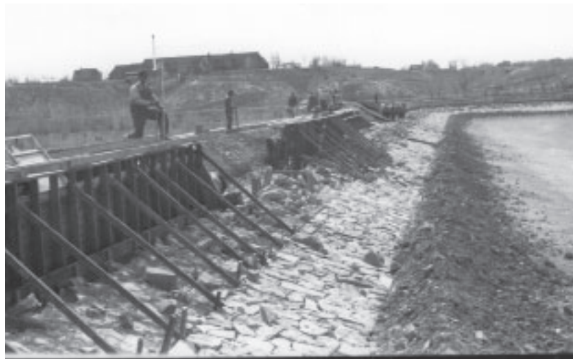
Water treatment settling pond under construction
