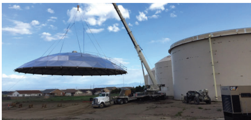
Jones Tank No. 1 gets a new roof
