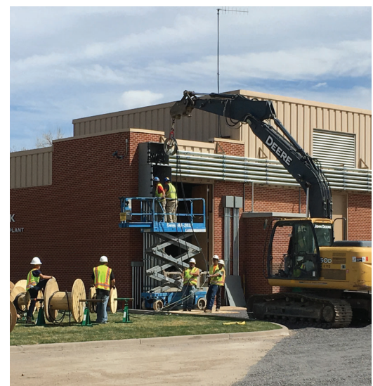
Upgrades at the Whitlock Treatment Plant
