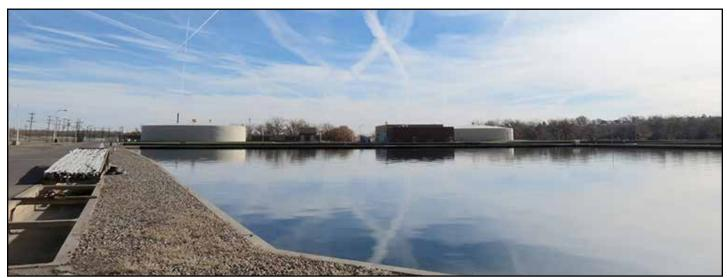
Sedimentation basin and storage tanks at Whitlock Water Treatment Plant
