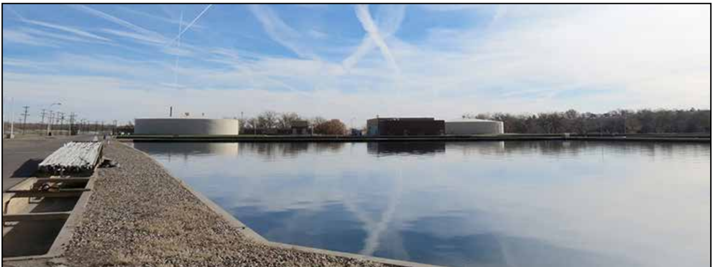
Sedimentation basin and storage tanks at Whitlock Water Treatment Plant
